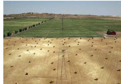
One \pm 500 kV bipole 150-200 foot ROW
