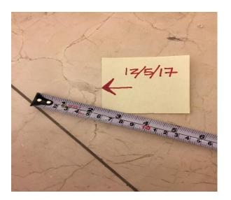
OFPM contracted with Lardner Monuments to make 14 repairs in late December 2017 and early January 2018. Those repairs addressed the worst areas and we haven't had to make additional repairs since. Each repair cost \$100 and involved a colored epoxy material injection.
