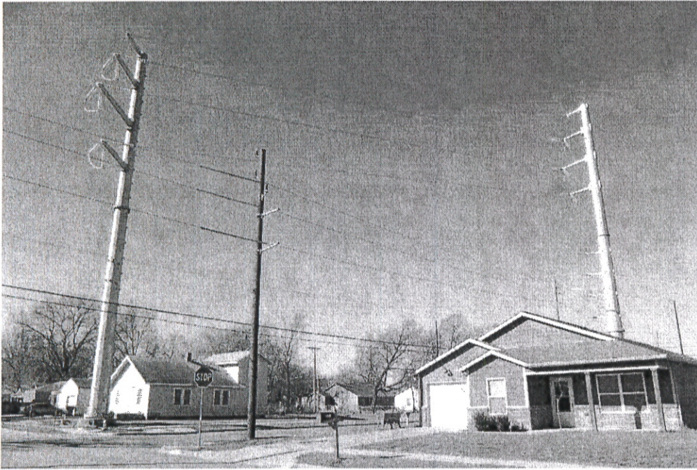
Top: Transmission tower (far left/far right) note relationship to blue Habitat home; though neither is “on” the 50 X 150 foot (7500 sf) property. Front yard set backs are 25 feet; concrete pad circumference 27’, 9’ diameter ).
